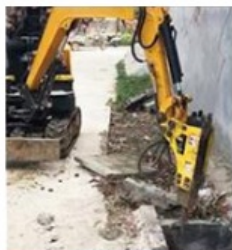
Crushing and demolition
