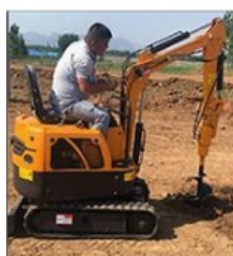
Rotary drill pits
