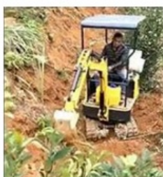
Digging a trench in the orchard
