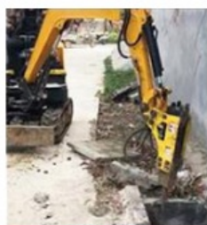
Crushing and demolition
