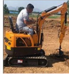
Rotary drill pits
