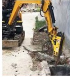
Crushing and demolition
