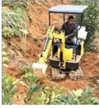
Digging a trench in the orchard
