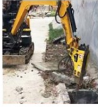
Crushing and demolition
